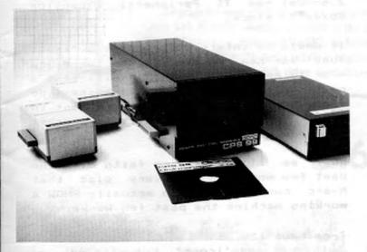
Great product #3 is their RS-232 card with 32k memory as well! (No, you can't use both the disk controller w/ 32k and this card at the same time!) This is totally TI compatible: 2 serial ports and one parallel port. The only difference is that the parallel port is NOT bi-directional like TI's. Price is estimated at about \$175.00 (US)
